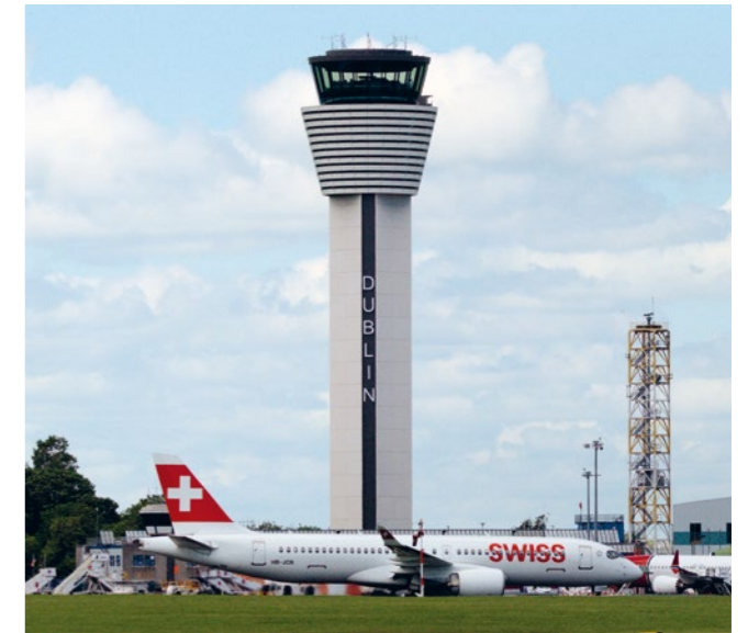
Tilger im Airport Tower Dublin
