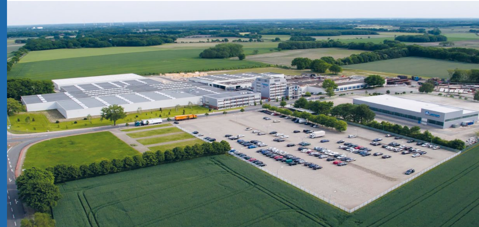
Aerial view of LISEGA headquarters in Zeven, Germany. The company, which was founded in 1964 in Hamburg, has been located here since 1971.
